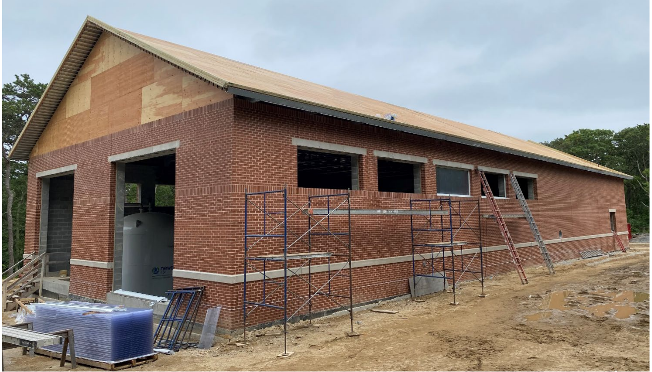
Wells 5 & 8 Treatment Plant – Roof Construction
