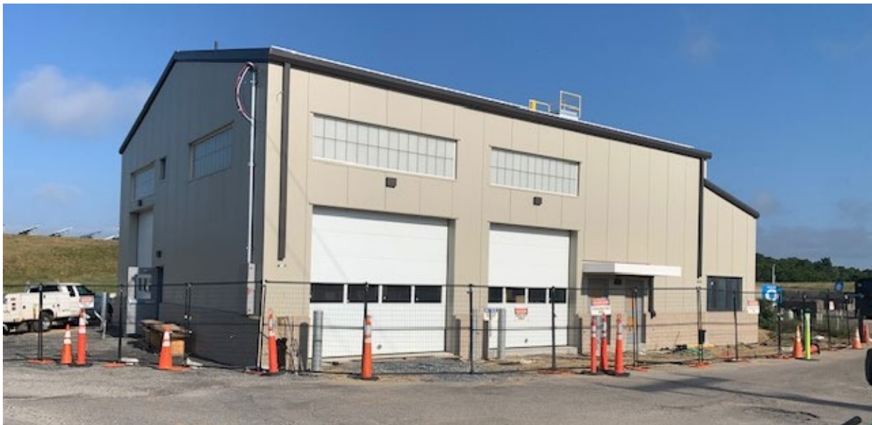
Building Envelope Construction at Transfer Station – Phase II (Priority I)
