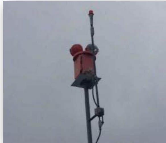
Figure 2-16: Non-Directional Beacon
