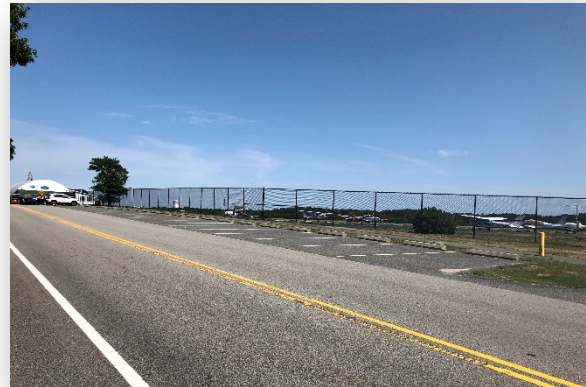
Figure 2-19: Parking on George Ryder Road
