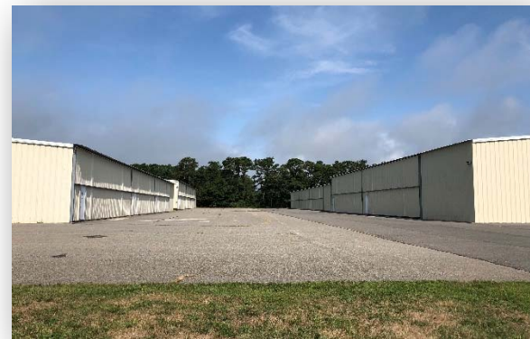
Figure 2-9: Nested T-Hangar Buildings
