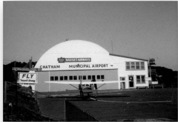
Figure 3-7: Historical Photo of Chatham Hangar Building
